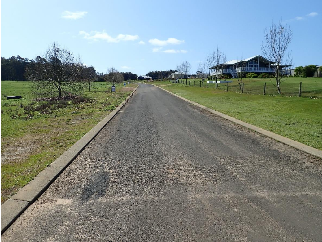
Figure 1: Photograph of the bitumen road, Lakeview Crescent.
