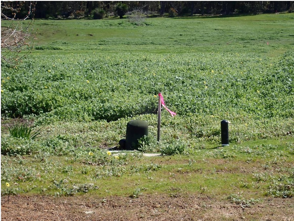
Figure 2: Photograph of the water and power supply on the lots.
