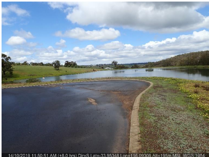
14/10/2019 11:50:51 AM (+8.0 hrs) Dir=S Lat=-33.95348 Lon=116.09308 Alt=195m MSL WGS 1984 Photo ID: Photo 1 Looking at the road reserve and dam.
